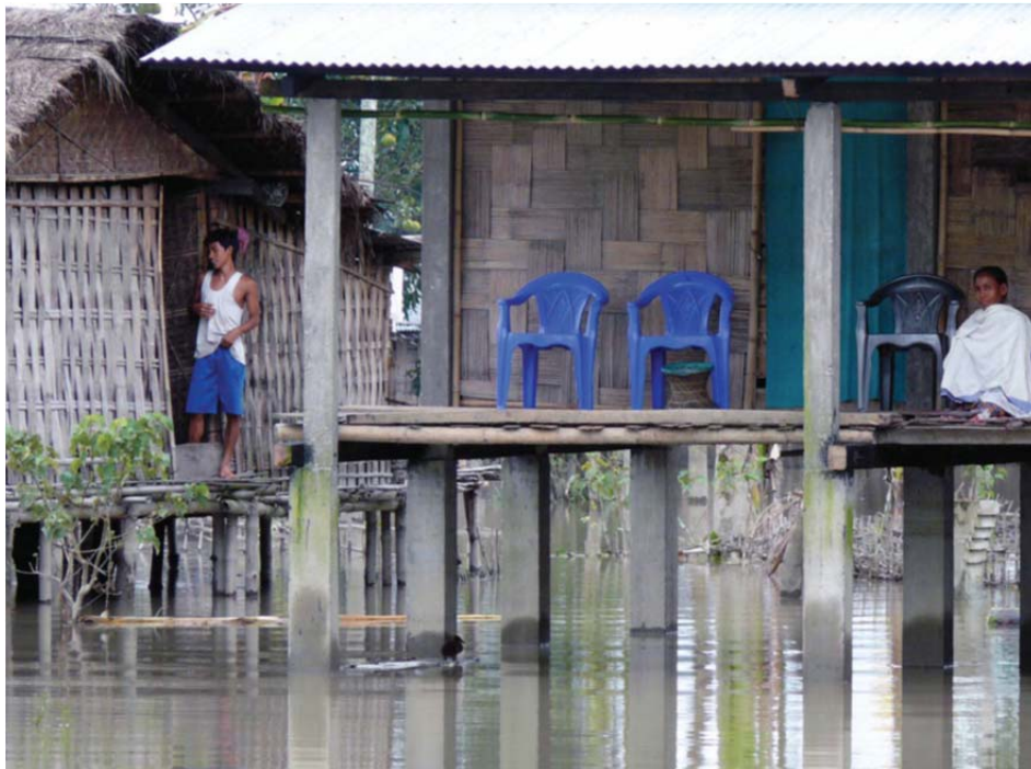
Figure 5. Chang-ghar (Mishing community, Nepal): left, original design of bamboo and wood; right, wealthier households invest higher stilts made of concrete
